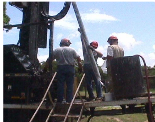
Figure 11. Rotosonic drilling can provide continuous soil and rock cores
